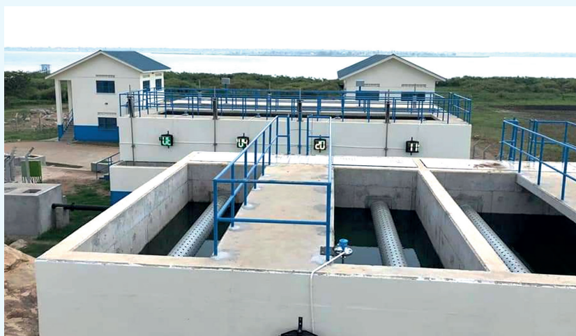
^^^The newly constructed Pallisa Water Supply and sanitation system
