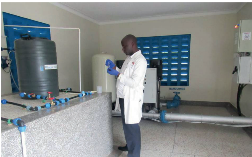
^^^Ensuring that the water quality consumed by the public is up to the required standards
