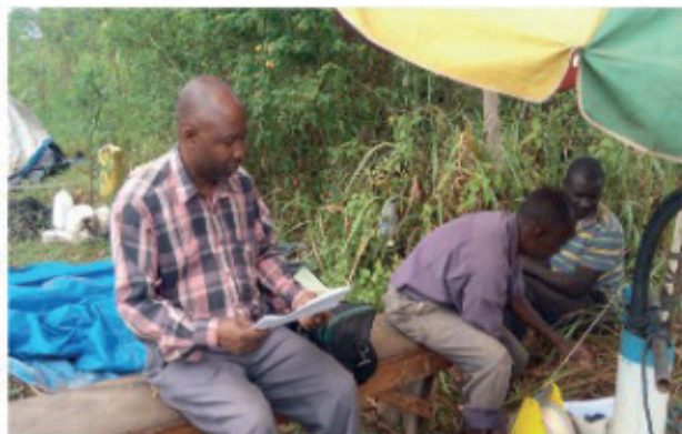
Measurements during test pumping the borehole
