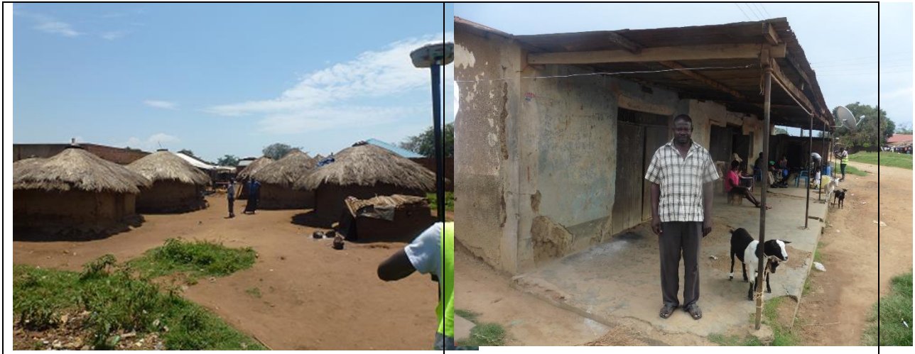
Plate 6-1: Some structures likely to be affected in Biko village
