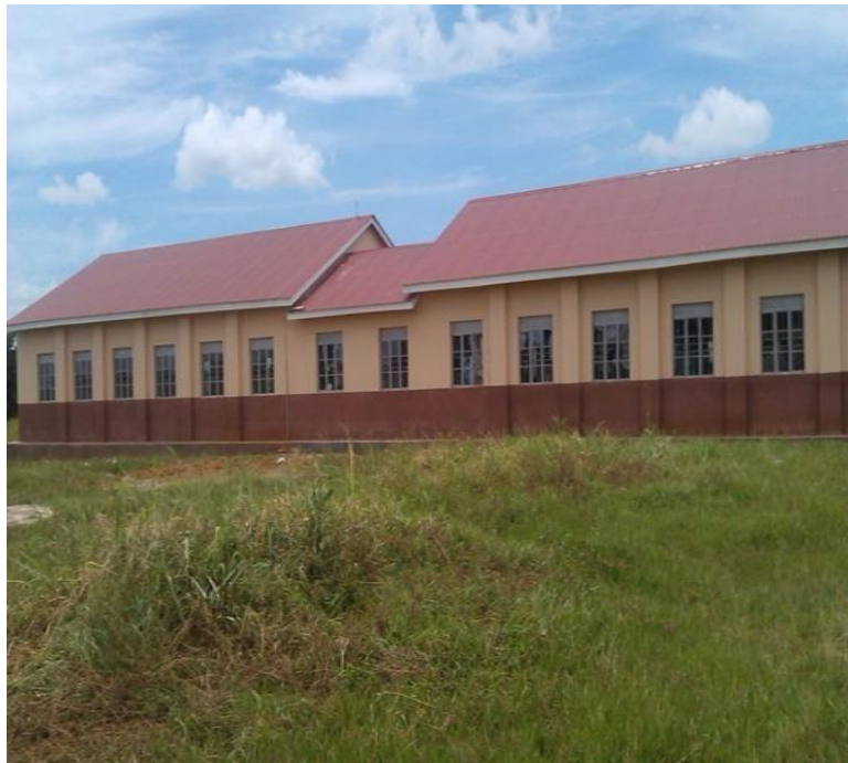
Figure 13: Some of the classrooms and staff house constructed in MFNP
