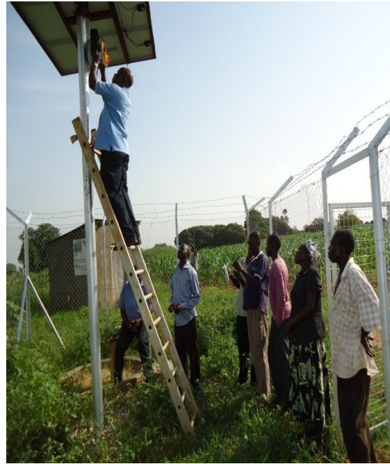
Timely electro mechanical repair works in schemes
