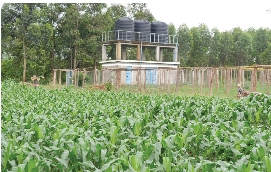
Reservoir tanks supply water to the gardens
