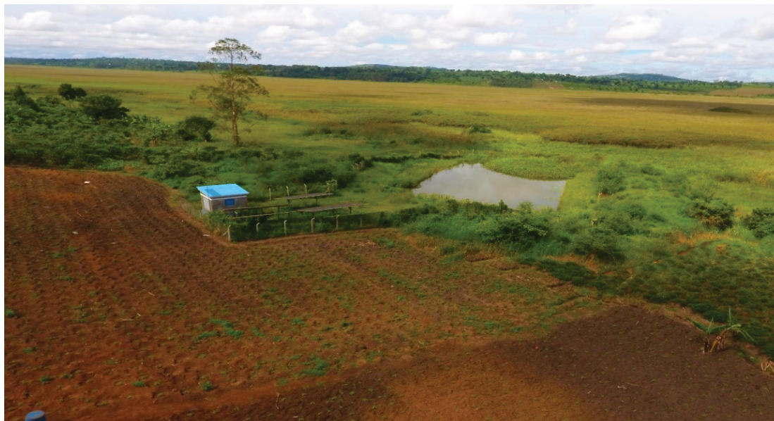
Water source (Nabafuzi swamp in Busoga village), a pump house, solar panels and gardens supplied with water for irrigation
