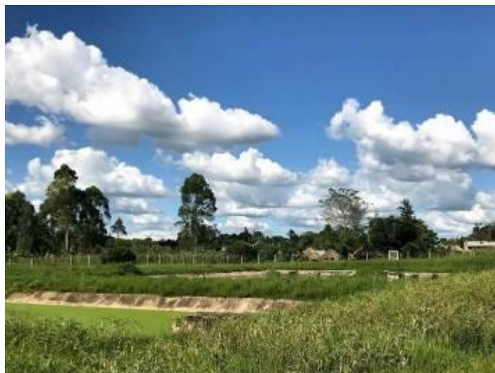
Figure 5-18: Waste Stabilization Ponds at Kiryandongo Hospital
