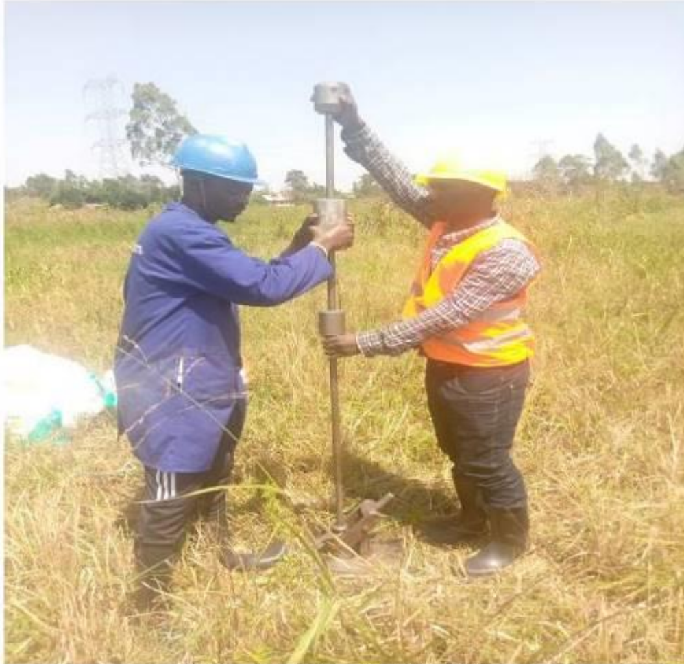
Figure 6: Conducting of the DPL test at site
