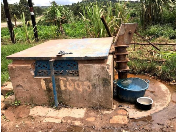
Borehole fitted with a handpump in Kagombe Village, Kibaale TC
