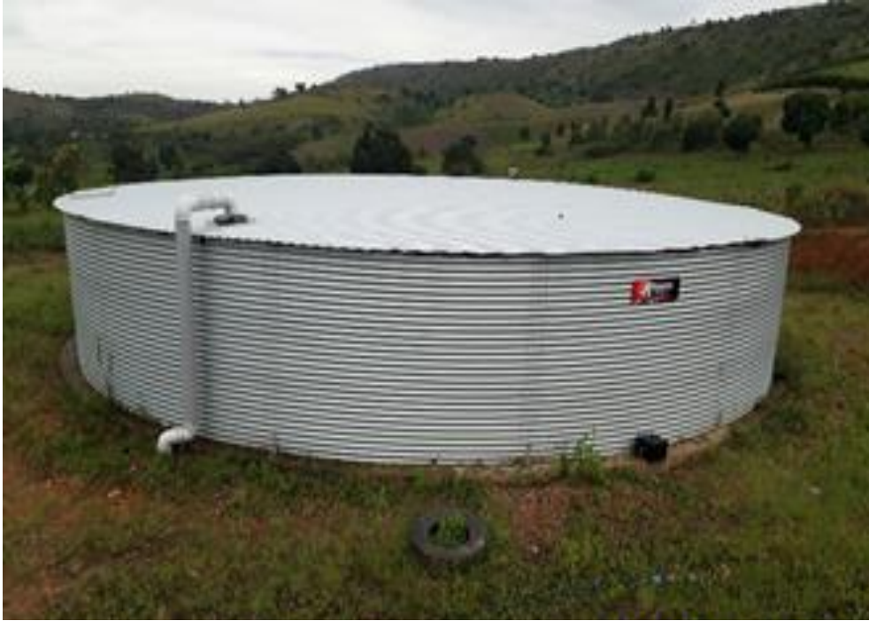
Figure 2-6: Rainwater Harvesting at Nsese Primary School, Nsese Village, Kifamba Sub - County
