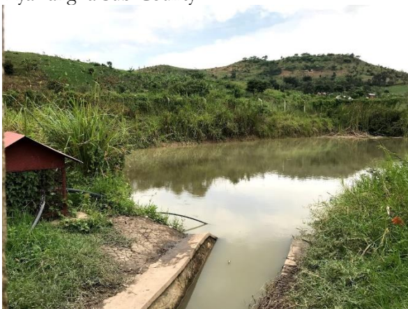
Dam in Kyakasenene village, Kibaale TC
