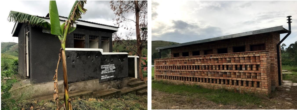
Lined Pit Latrines at Education Institutions in Kibaale TC Figure 2-7: Sanitation Facilities in Kibaale TC
