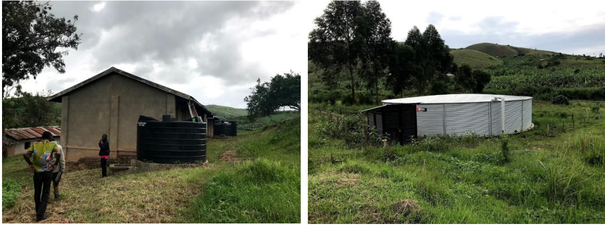
Figure 2-3: Rainwater Harvesting at Institutions in Kyakasenene village, Kibaale TC
