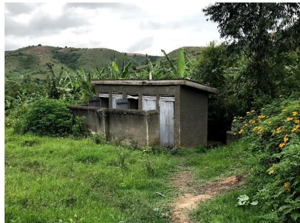
Unlined pit latrine at school in Tolero Village, Kibaale TC
