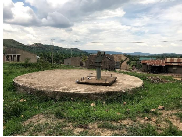
Shallow well fitted with a handpump in Kyalulangira Village, Kyalulangira Sub-County
