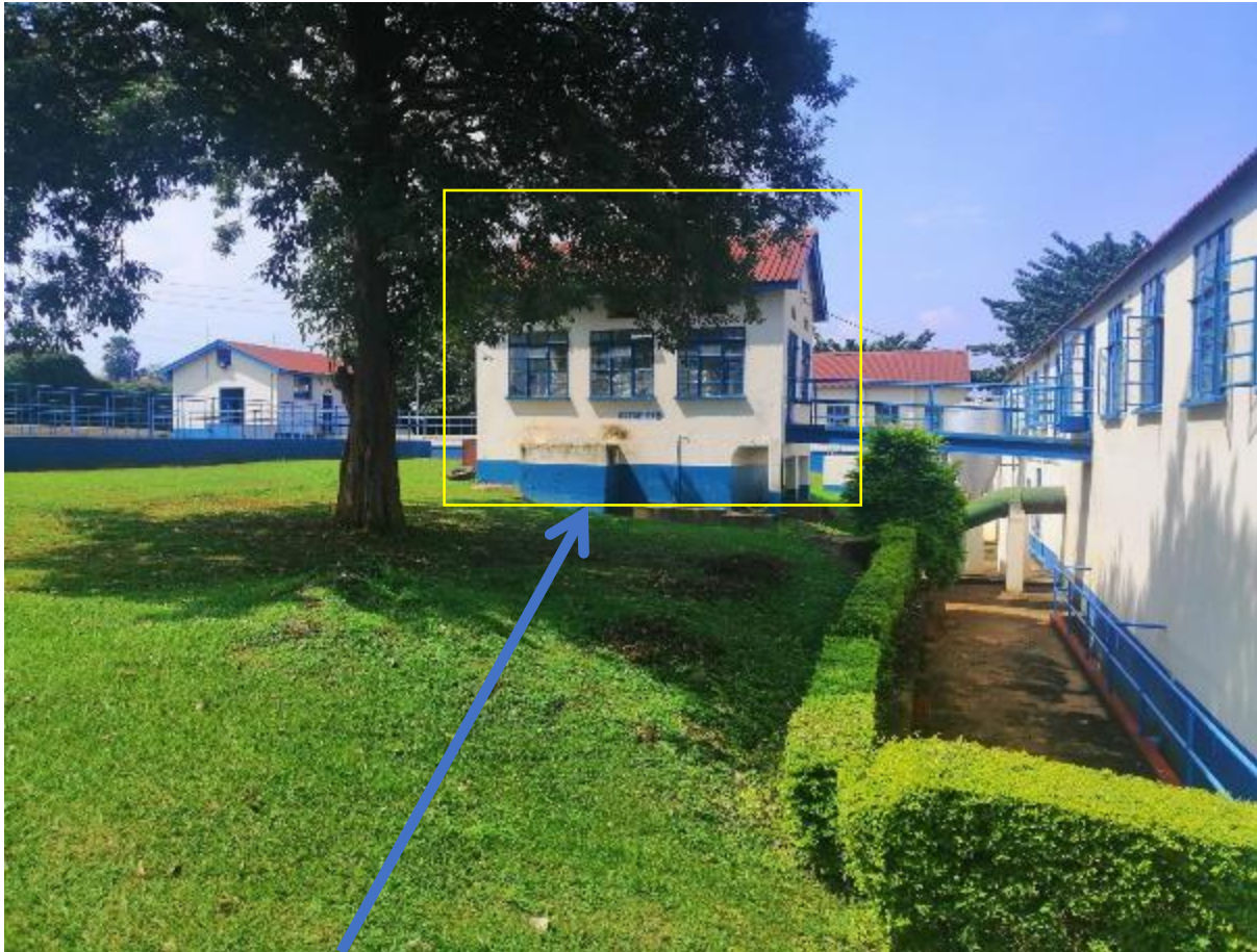
Plate 4.25: The structure that will be affected by the construction activities
