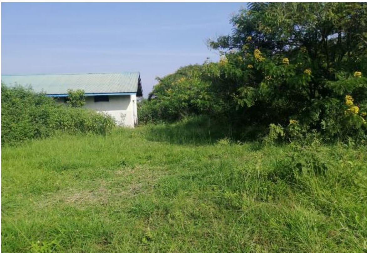
Plate 4.30: A pump house, the bushy part is the site where the incomplete tank structure is located
