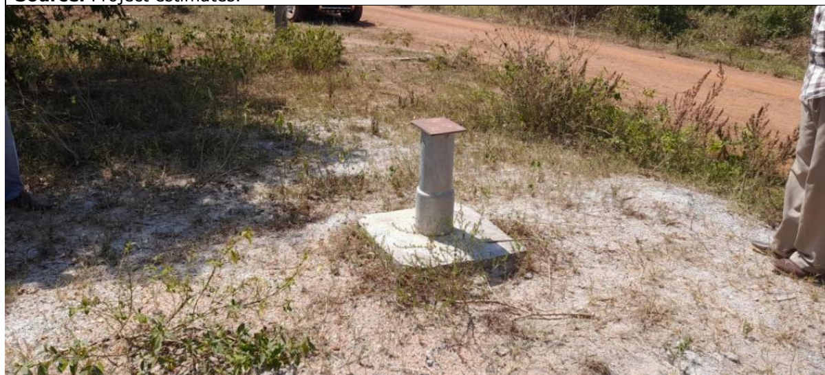
Plate 1: The Itek Village Borehole (DWD 79457) in Itek Parish, Itek Sub County.
