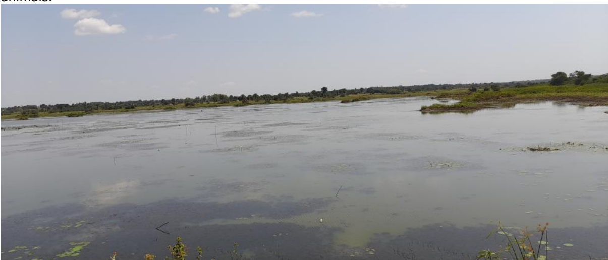
Plate 16: One of the constructed dams in Itek village in Barr RGC
