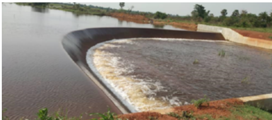
Present structure of the spillway at Tochi with flowing water ■
