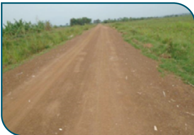
Access road at Dobo II irrigation scheme ■
