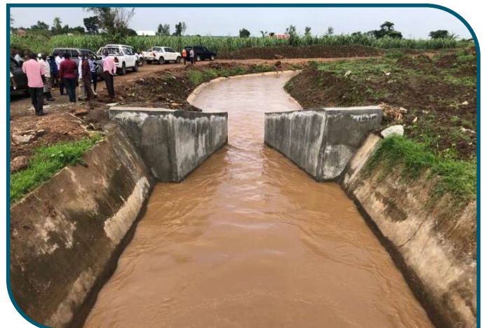
A view from an upstream side of an entry into the main canal at Dobo II irrigation scheme, Butaleja district ■
