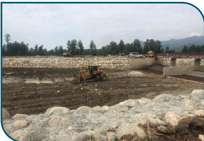
Cleaning of the channel bed downstream the weir ■
