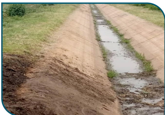
Secondary canal being cleaned to receive water at Mubuku II irrigation scheme ■
