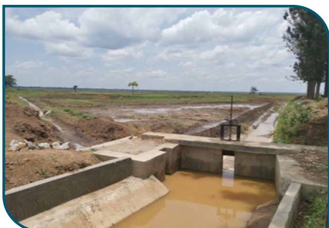
Completed head regulator at Doho irrigation scheme, Butaleja district ■
