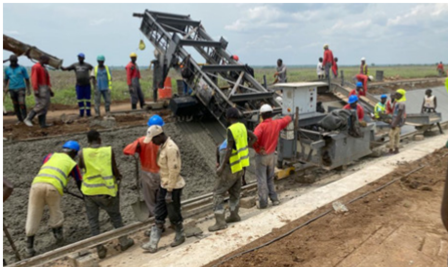
Concrete lining of water canal at Wadelai irrigation scheme ■
