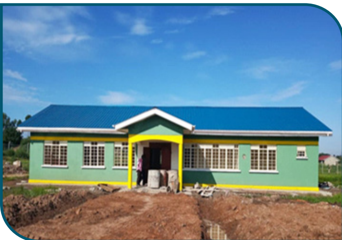
One of the scheme buildings at Tochii irrigation scheme, Oyam district
