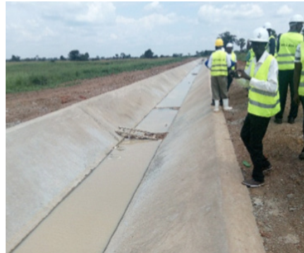
Completed concrete lining of main canal at Doho II irrigation scheme, Butaleja district
