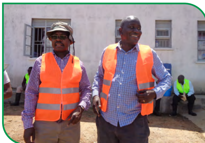
Mr. Pius Wakabi, PS –MAAIF and Mr. Alfred Okidi, PS – MWE preparing for field inspection at Wadelai irrigation scheme, Pakwach district ■
