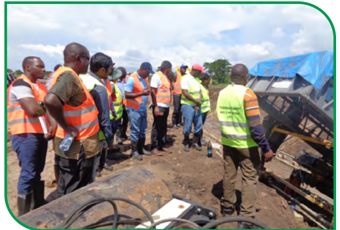
Members of FIEFOC 2 Project Steering Committee inspecting ongoing construction work of canals using advance machines at Wadelai irrigation scheme, Pakwach district ■
