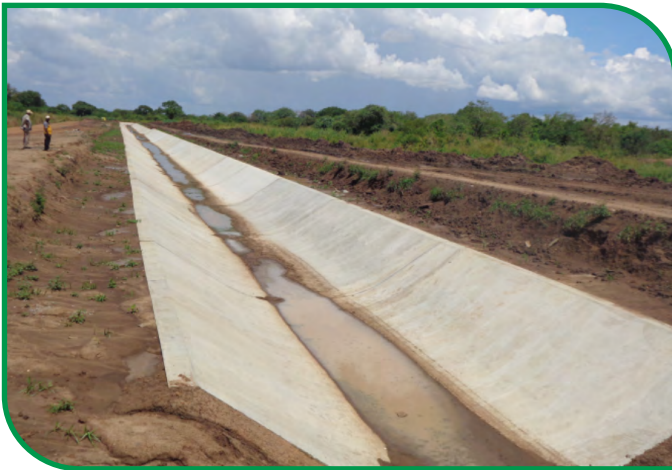
One of five secondary canals under construction at Wadelai irrigation scheme in Pakwach district ■
