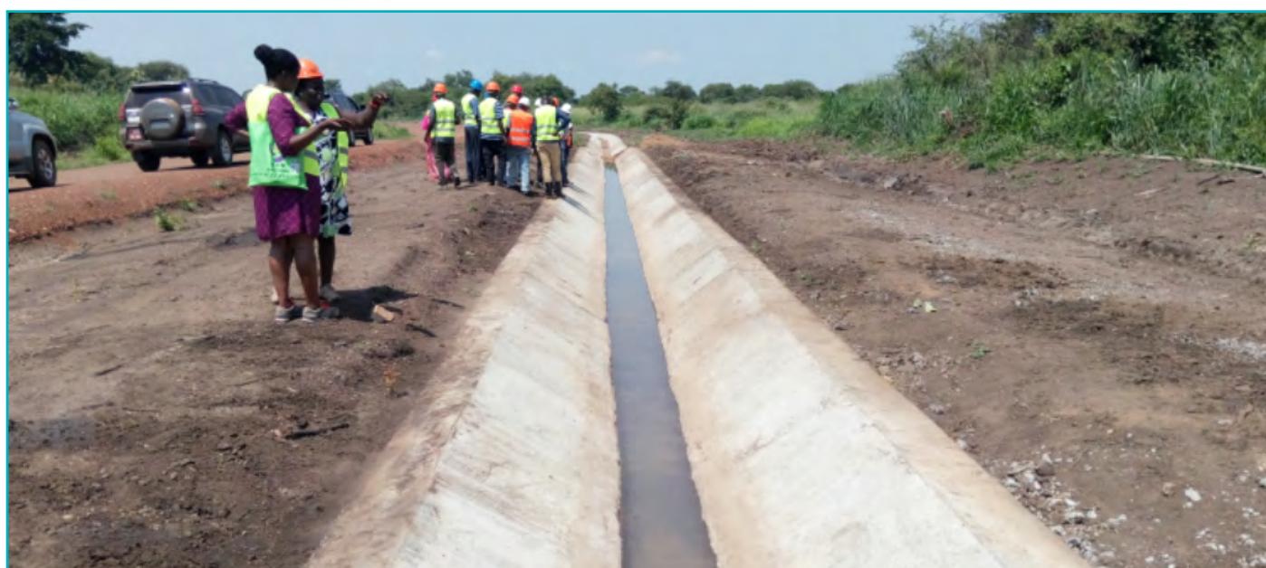
One of the secondary canals completed at Wadelai irrigation scheme, Pakwach district ■
