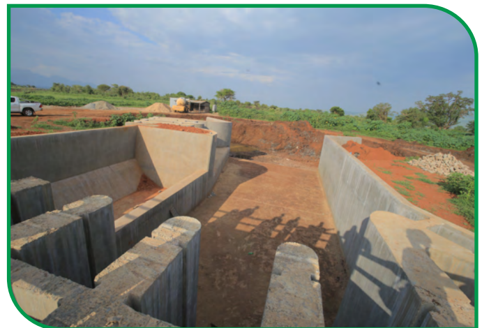
Kabajiria headworks under construction at Ngenge irrigation scheme, Kween district ■
