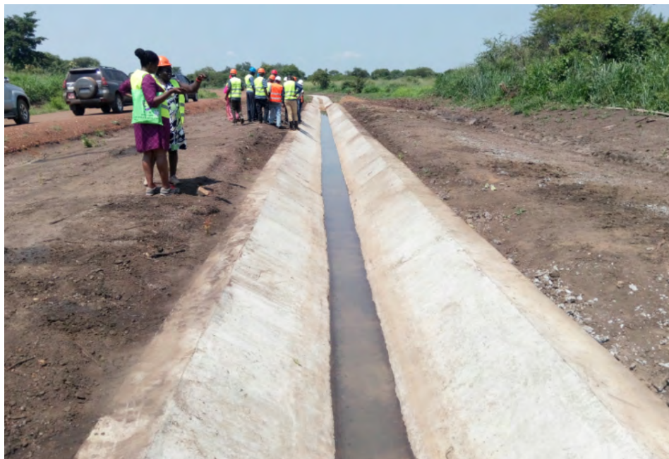
ADB mission inspecting one of the completed secondary canal at Wadelai irrigation scheme ■
