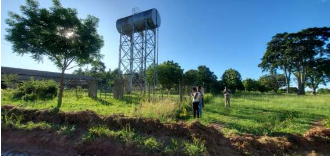
Figure 2-17: Existing tank for Kasilo (36N 0539088 0171895) which will be used for Kasilo
