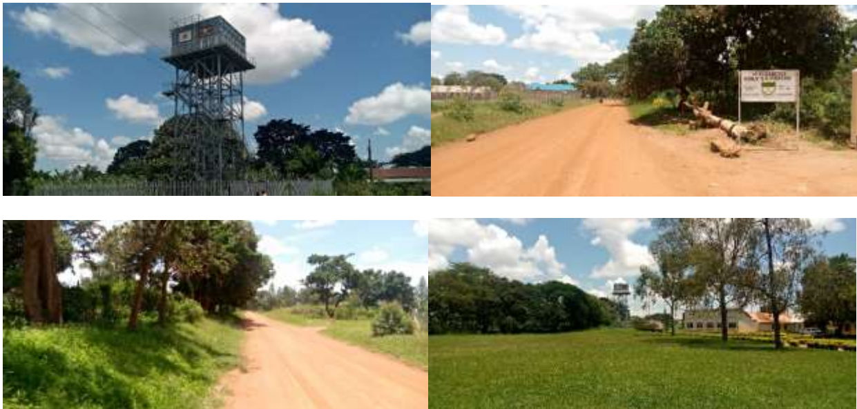
Figure 2-16: Showing the access route where piped water system will pass, the tank in Kidetok Town Council, Serere District.
