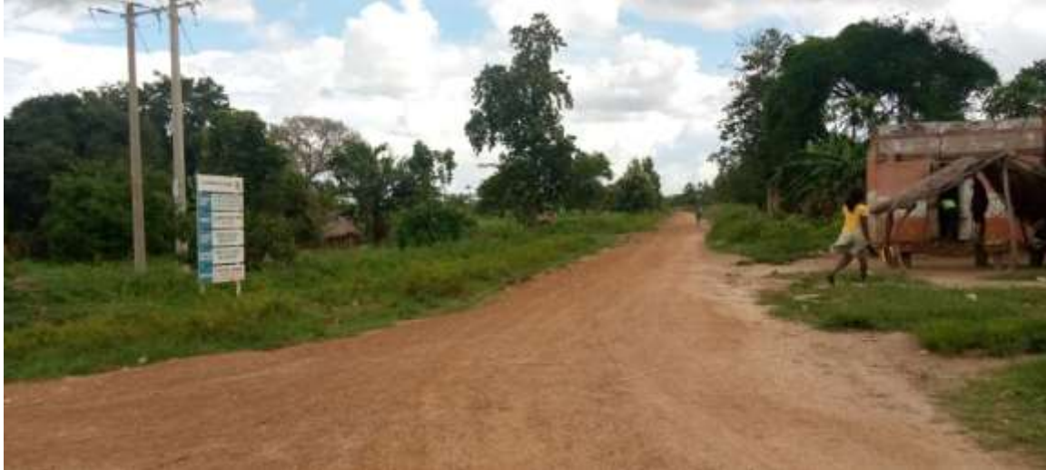
Figure 2-9: Showing access route where piped water will pass.
