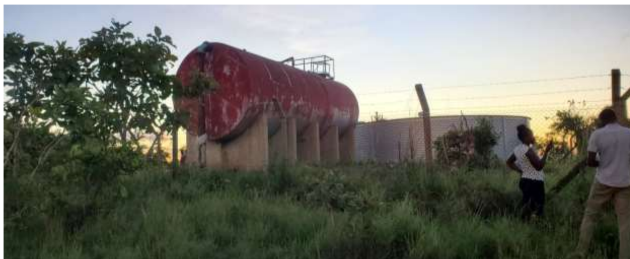
Figure 2-20: Existing tanks at Kikota Hill in Serere Town Council where the water reservoir will be installed
