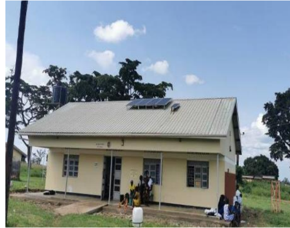
Solar Panels at Cwero HC III
