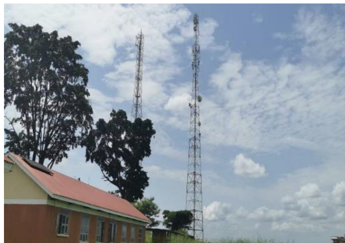
Plate 9: Communication System - Masts in the project area. Taken by the Sociologist, March 2023
