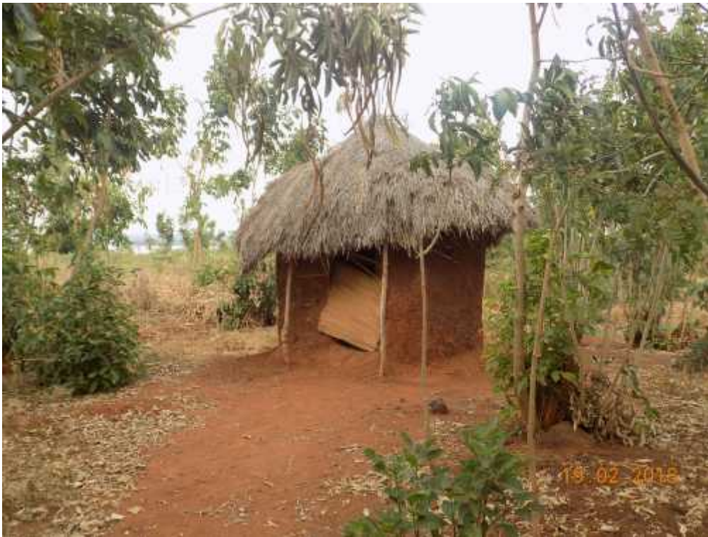
Picture 4-5: Example of pit latrines in project area
